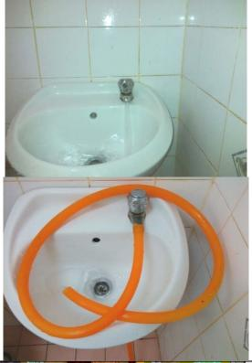
3h. For places where it is difficult to access, open the tap at the speed you want to measure and connect it with a hose. This way you can still measure the time taken to fill up 1.5 litre of water.
